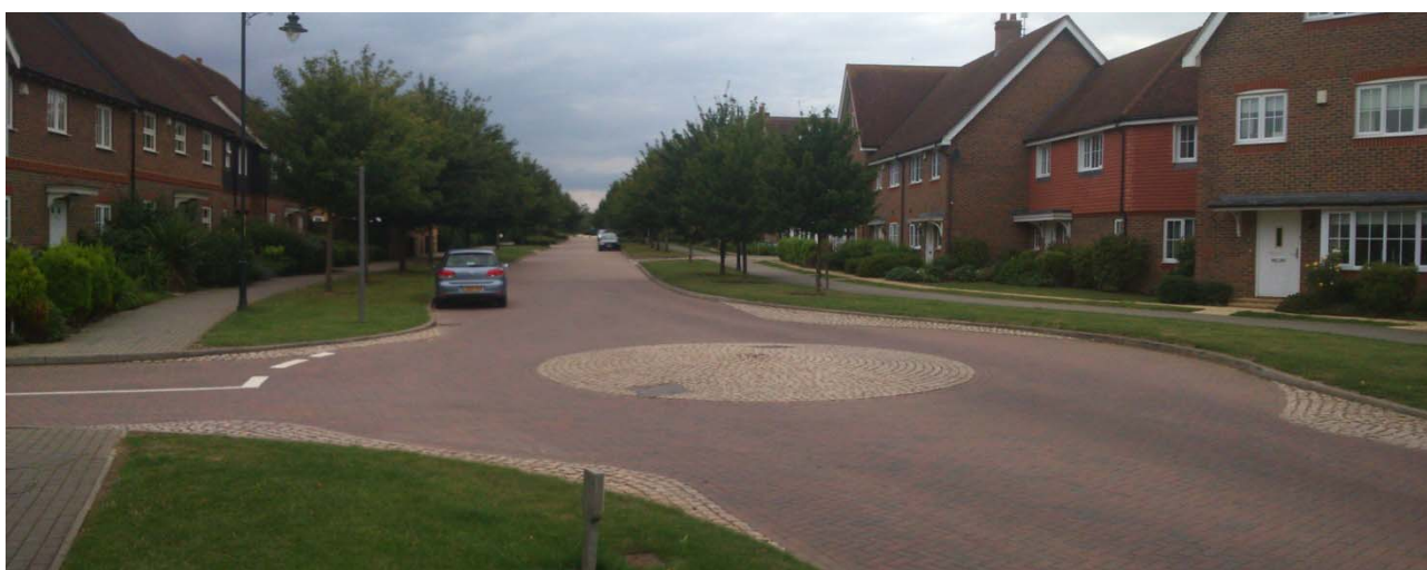
Fig. 6: West Malling, Kings Hill - spine road lozenge and overrun feature calms traffic by occasional introduction of a feature obstacle. These should be tracked for 12m buses.
