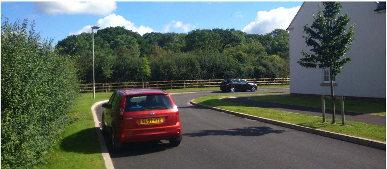
Fig. 3: Tight bends and limited visibility, combined with 6m width and uncontrolled on street parking means this road is not suitable for bus operation.
