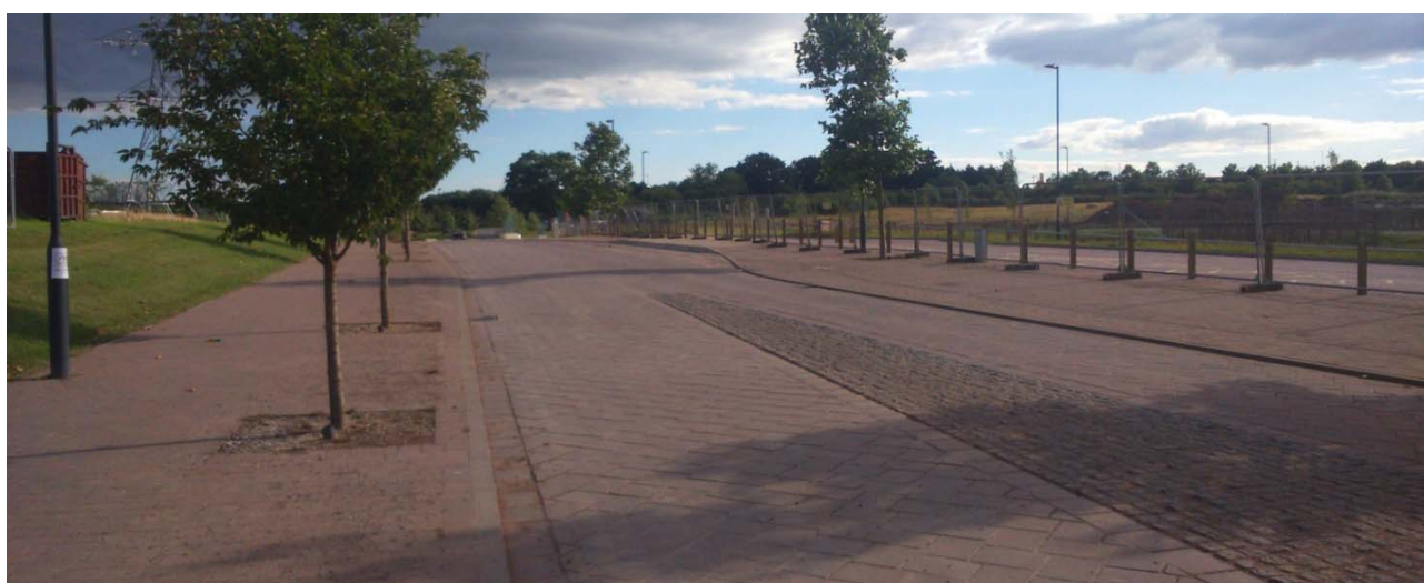
Fig 9: Bristol Lyde Green Spine Road – approach to surface treatment appears to narrow the carriageway, while allowing for tracking of larger vehicles.
