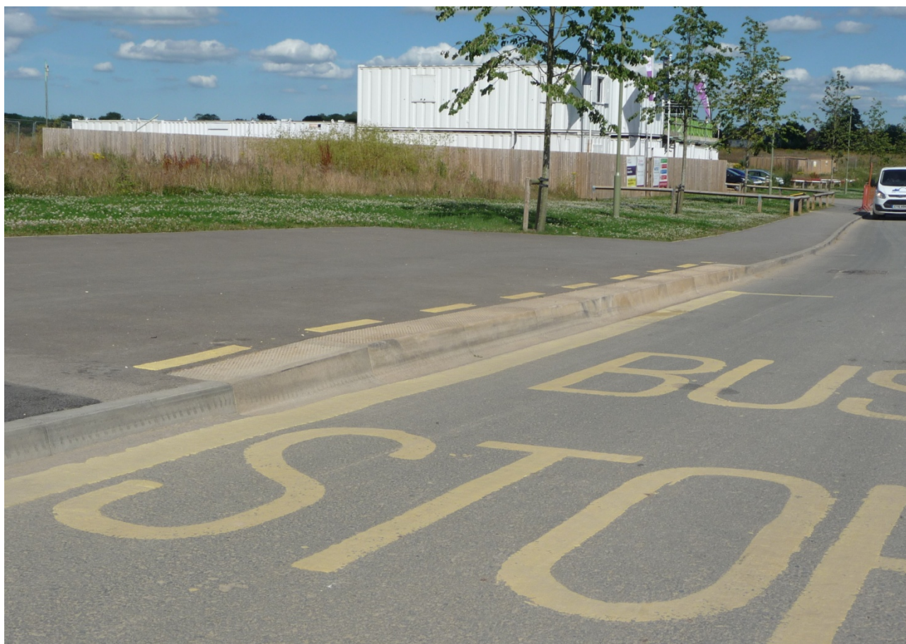
Fig. 31: Andover, East Anton MDA- preferred raised boarder detail.
