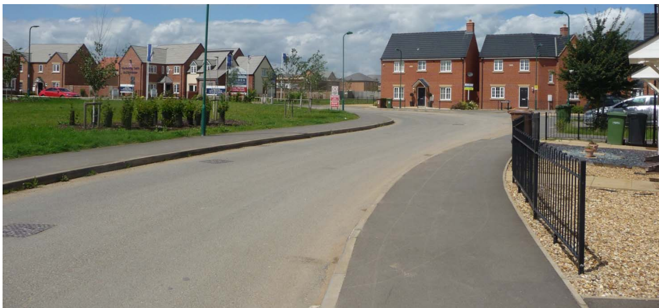
Fig 4. Peterborough, Cardea. Appropriate road curvature reduces speed without an excessively tortuous alignment.
