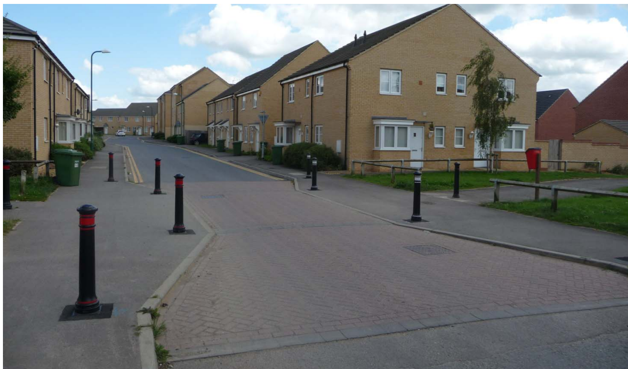
Fig. 8: Peterborough, Cardea - short single-track throttle at pedestrian crossing. Note the gentle ramp transition and good cross-visibility.
