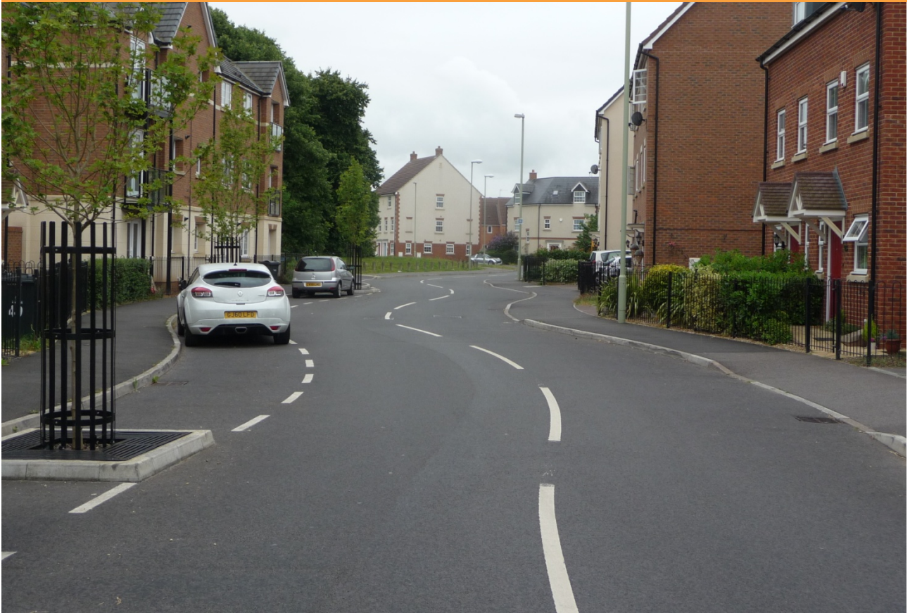
Fig 2: Unnecessary deflection. This road was designed to accommodate buses but this has proved to be impractical. Just 2 or three cars parked on-street, would make tracking very difficult for buses.
