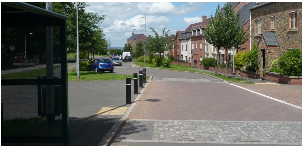
Fig.10: Telford Lawley ph 1 - careful use of offsets, changes in width and surface, and controlled on-street parking are used to create visual interest and reduce speeds while avoiding delay to buses.
